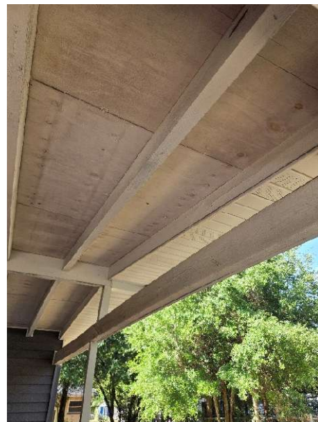
Porch Rafters & Beams Positive
