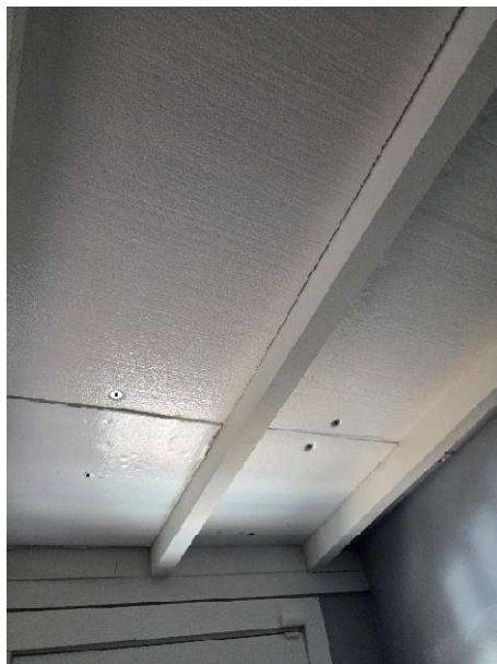
Typical Ceiling Rafters Positive
